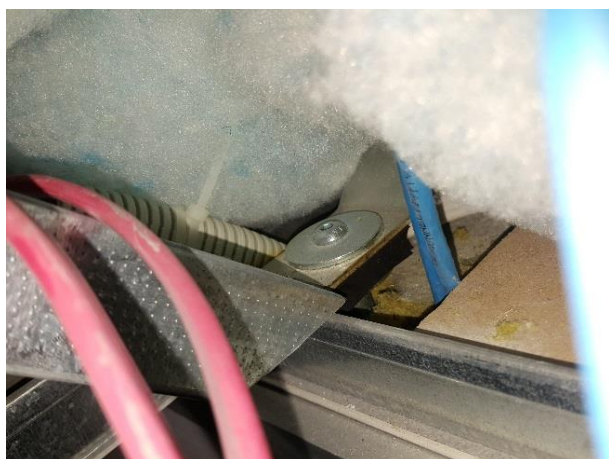
Track-lok bracing of partition walls
