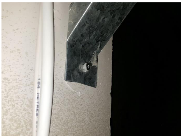
Partition wall bracing let down by fasteners 2
