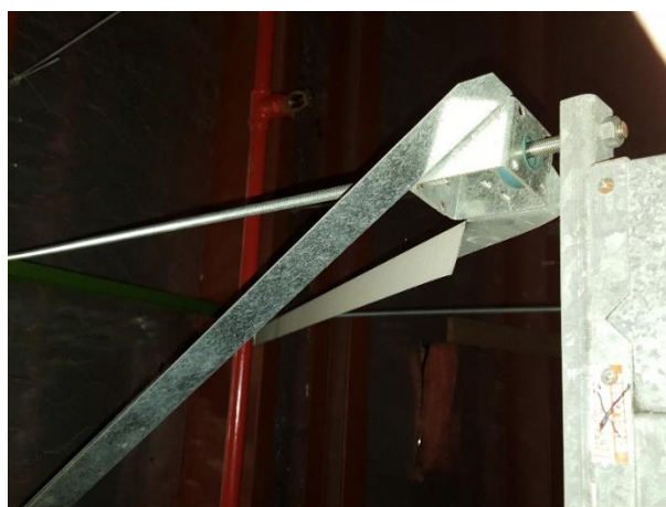
Air handling bracing let down by clearance, angle and general poor methodology
