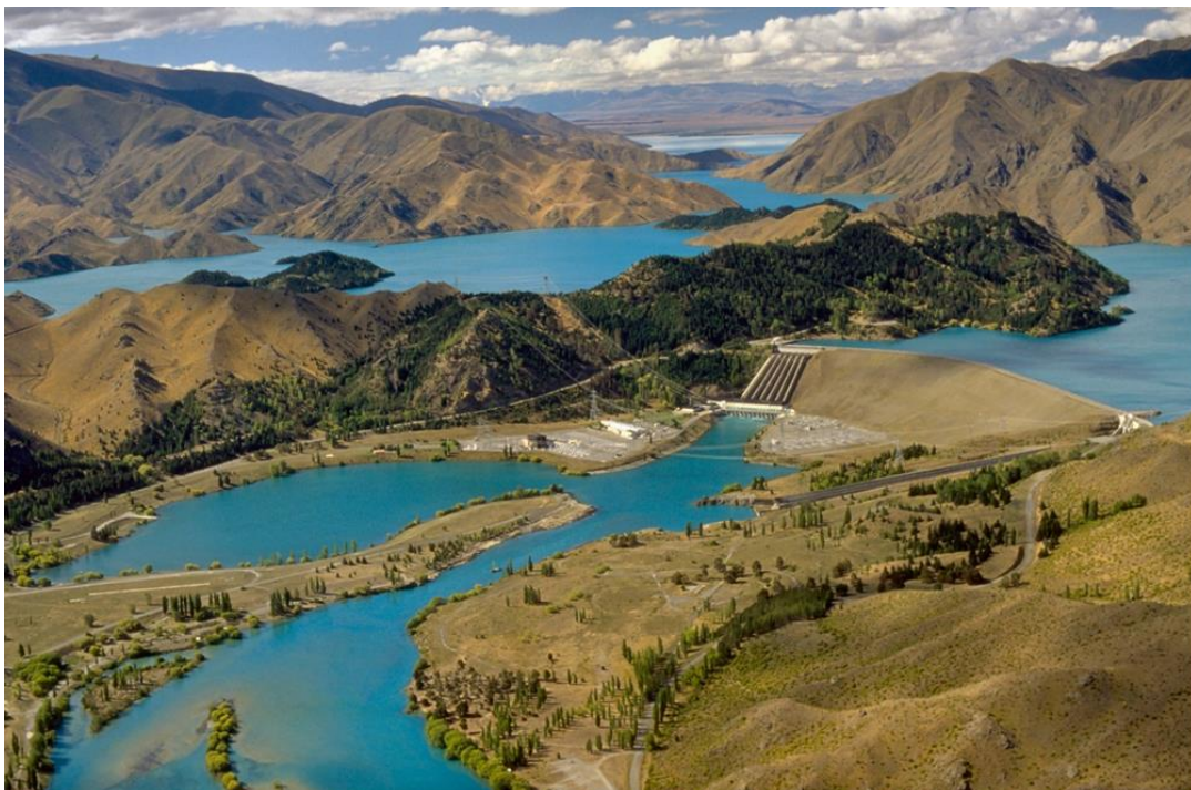
Benmore Hydro Power Station, Otago, South Island, NZ
