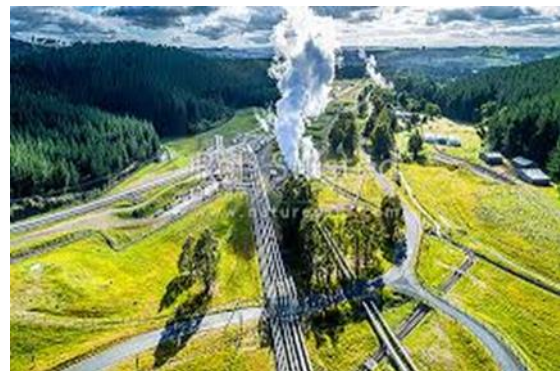
Geothermal Generation Plants
