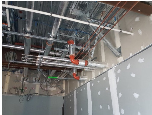
Figure 1: Seismic Restraints of Services
