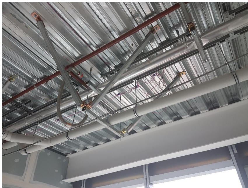
Figure 3: Seismic Restraint of services
