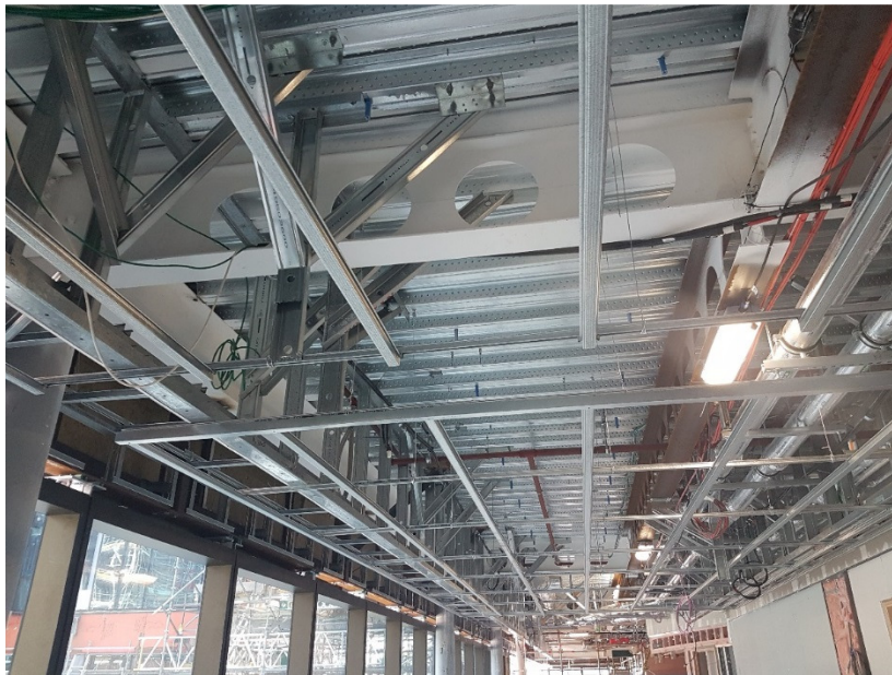
Figure 2: Seismic Restraint of Services and Ceilings
