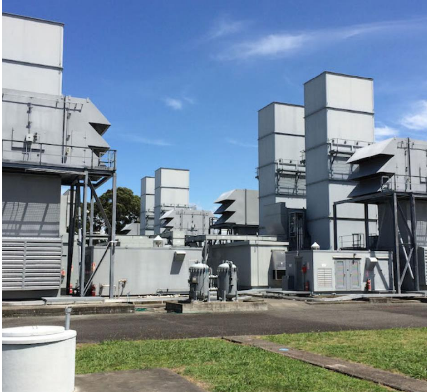
Whirinaki power station
