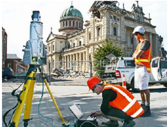
Laser scanning earthquake damage to the Christchurch Basilica.
