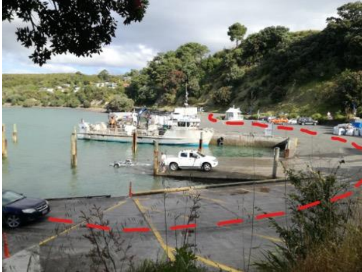
Picture 1. Recreational boat ramps in the foreground. Red dotted line indicates access route public users must take on hardstand, skirting around commercial operating zone. Source: Fraser Stobie, onsite December 2018.
