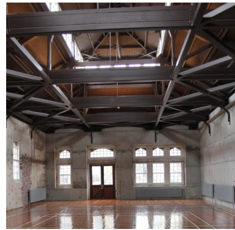
Figure 6. Steel bracing at eave level used to strengthen the Christchurch Arts Centre gymnasium
