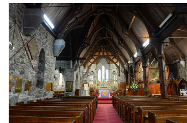
Figure 2. View of the Cathedral nave showing internal face stone walls and timber roof structure
