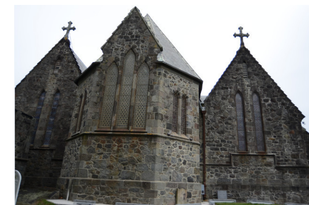
Figure 1. View of the Cathedral from the North-west elevation
