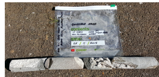
Figure 4. Stone wall core taken from East elevation of Taranaki Cathedral
