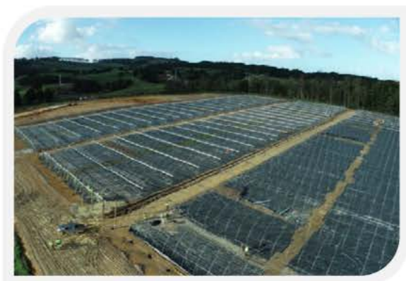
Figure 5: Construction of tunnel houses for horticulture
