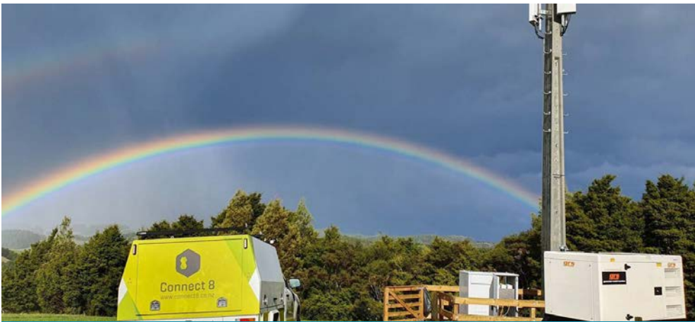
Te Arai Cell Tower – Tairāwhiti (photo taken from NZ Herald article)
