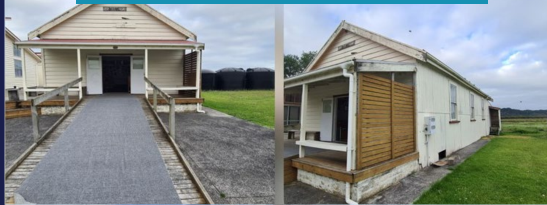
Mataitaua marae before renovation – Tai Tokerau / Northland
