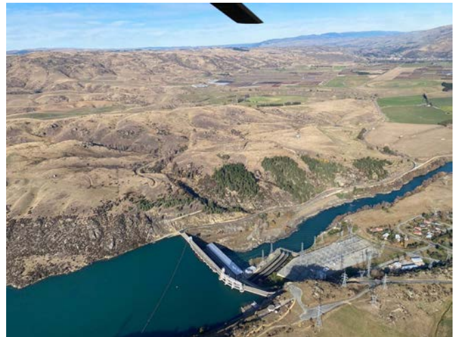
Photo 2: Roxburgh Dam and Teviot Valley beyond
