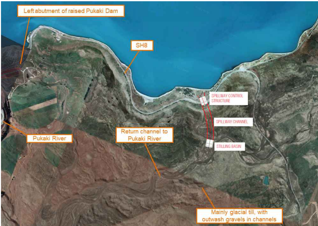
Figure 32 - Location of the proposed spillway at the left abutment of the existing dam
