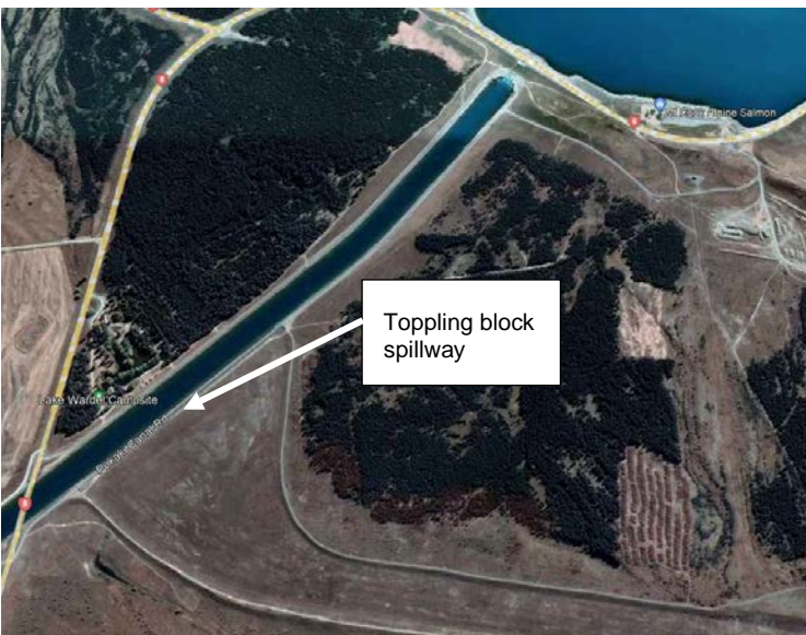
Photo 4 - Pukaki Canal Spillway
