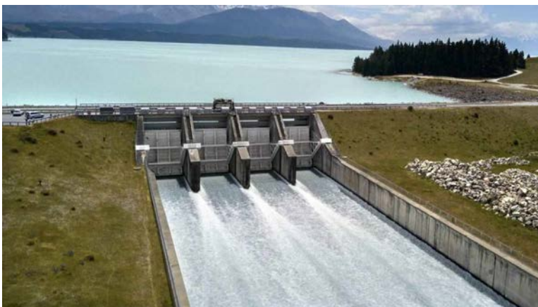
Photo 1 - Pukaki Spillway Gate
