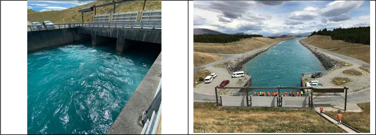
Photo 2 - Pukaki Canal Inlet Structure
