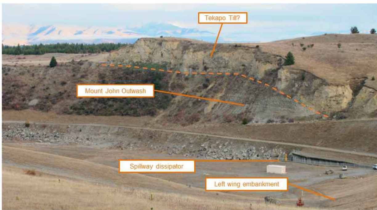
Figure 27 - Annotated image showing key geological units (modified from Barrell & Read 2013)
