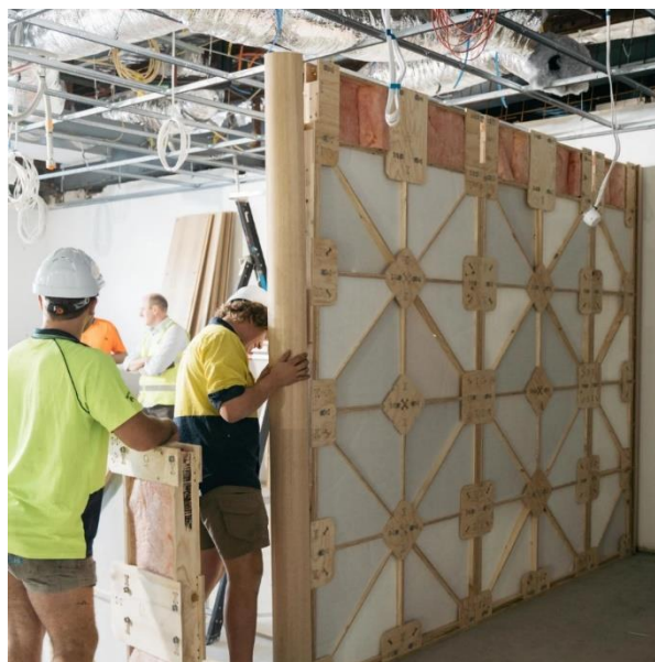
Figure 13: Example of the XFrame modular, deconstructable system. 81
