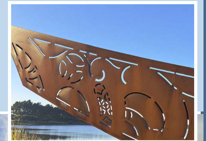
Mahi Toi designs associated with the pump station are integral to the wider Stead Street climate resilience project. The above image shows the design detailing at the end of the new sheet pile wall, conceptually transforming it into a Waka Tiwai.
