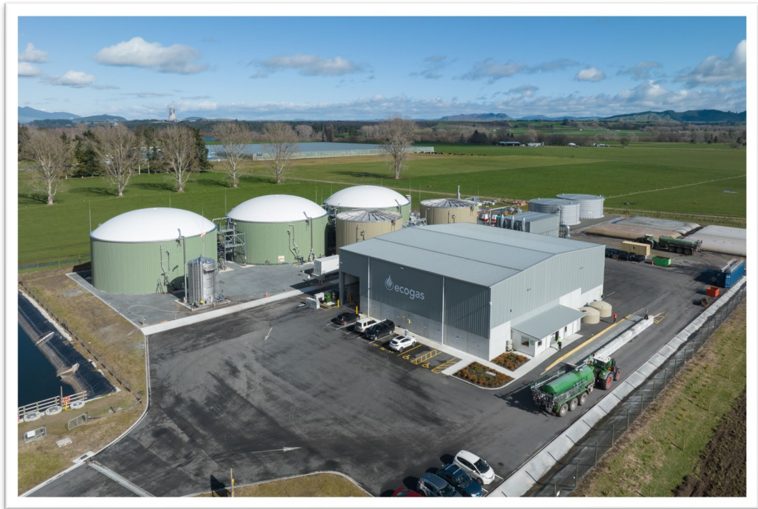
Ecogas Reporoa Organics Processing Facility
