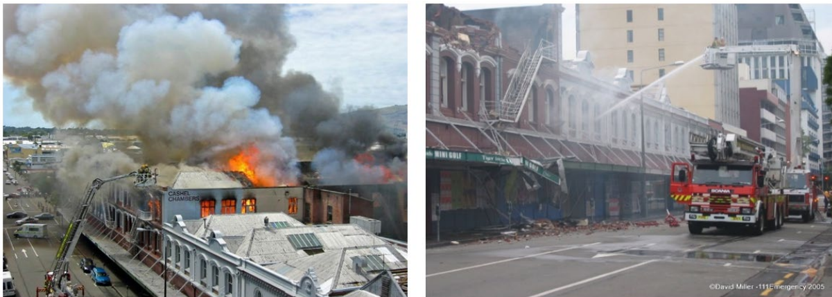
Figure 4. Cashel Chambers building in Christchurch – 23 January 2005 showing the fire and showing fallen debris on the road
