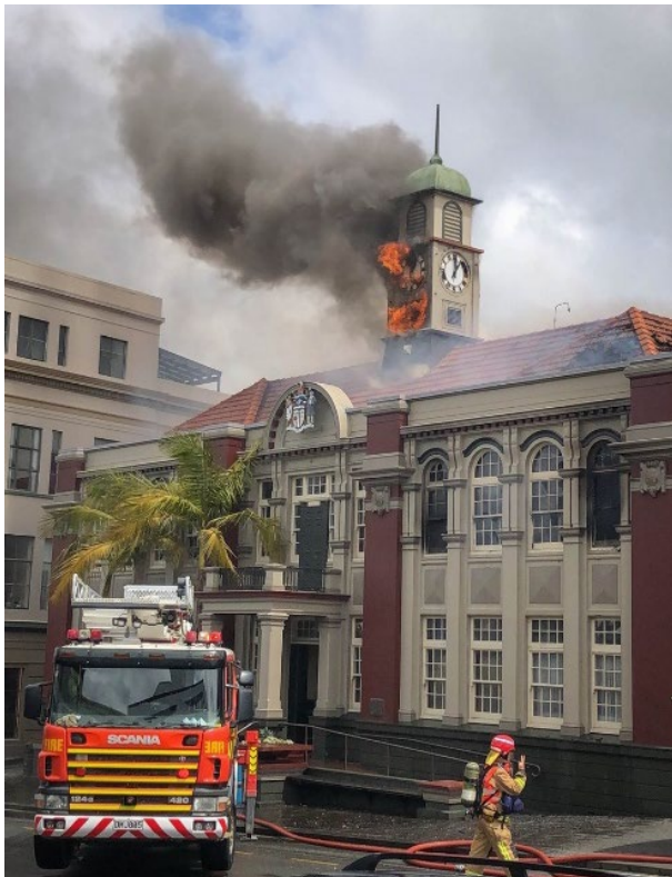
Figure 8. Whangarei Municipal Building – 20 October 2019
