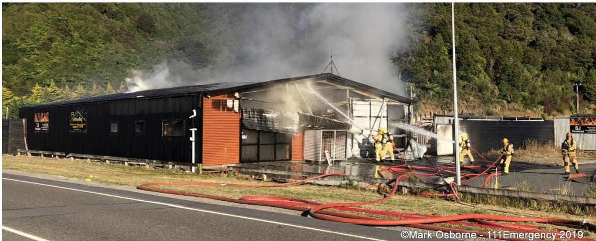
Figure 7. Roofing building – 25 January 2019
