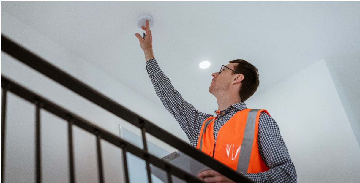
Figure 3. Specified systems such as emergency warning systems are subject to inspection, maintenance and reporting procedures under the Building Act
