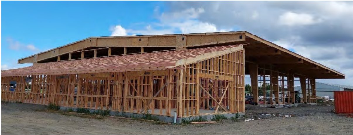
Construction for BBI Wood Processing facility, Hawke's Bay
