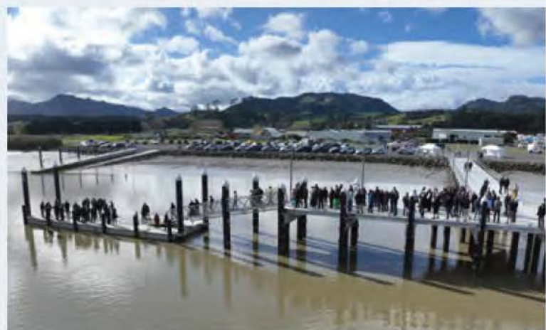
TOP: Kōpū Marine Precinct during construction
