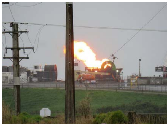
Right: OMV Pohokura production station, 14 June 2024 (photo by Abbie Jury).
