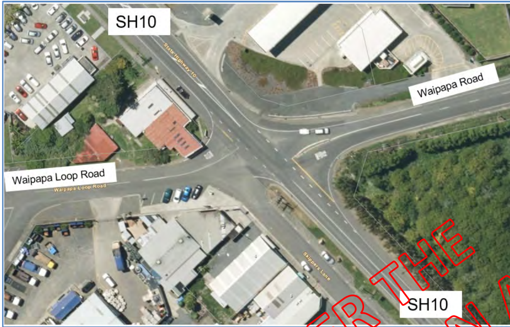
Figure 5: SH10 / Waipapa Road / Waipapa Loop Road Intersection (Source: Far North Maps)
