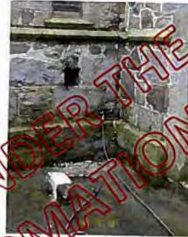
Figure 3. Stone block removed from external facade of Taranaki Cathedral
