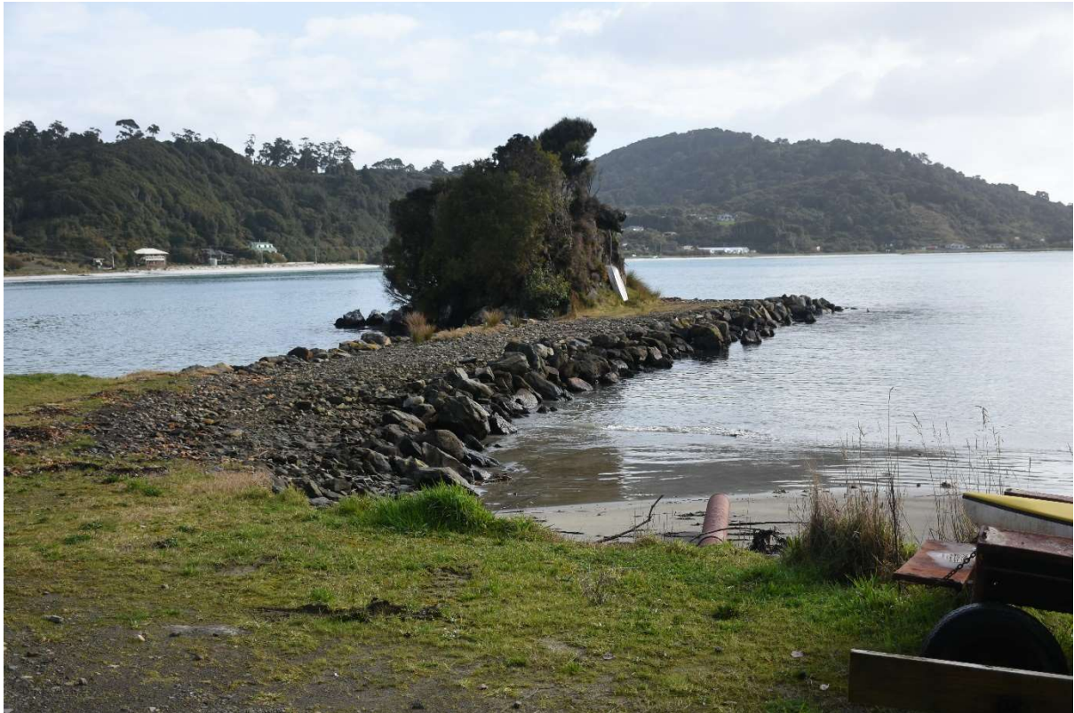
Site photo 9. Rockfill wharf. Possible landing site for barge.
