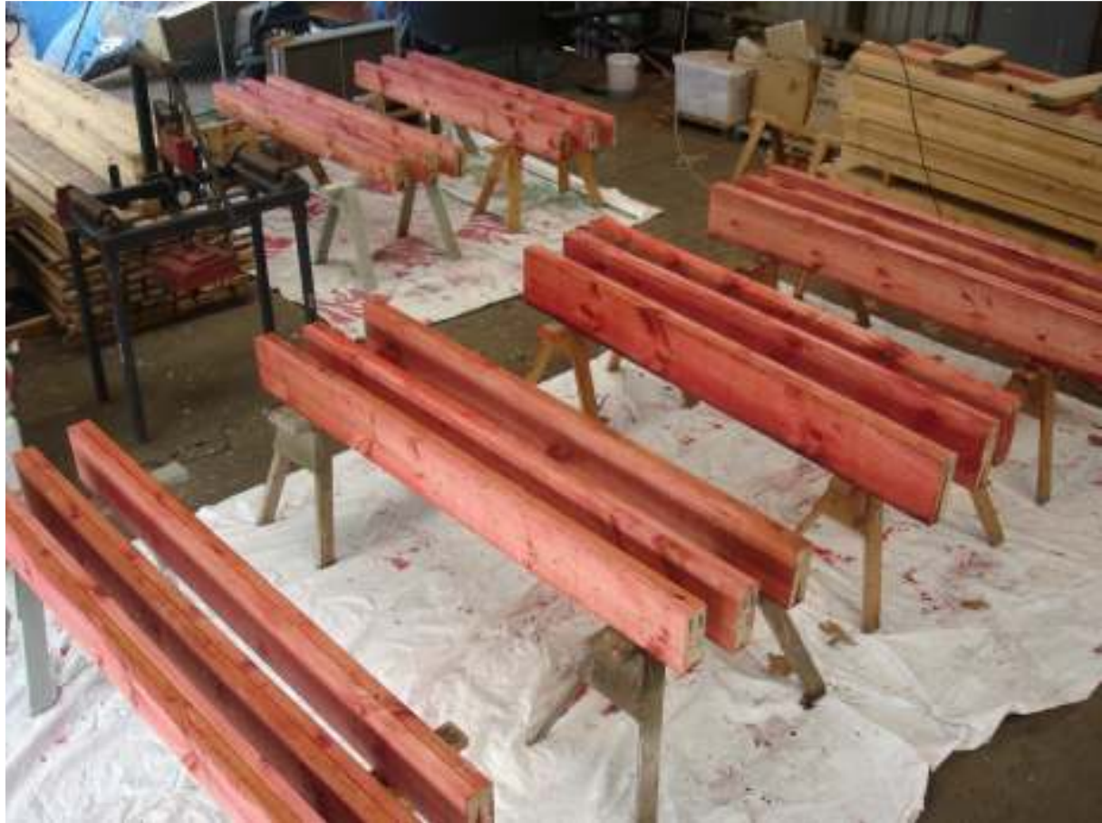
Figure 5: Lintels after injection and coating.
