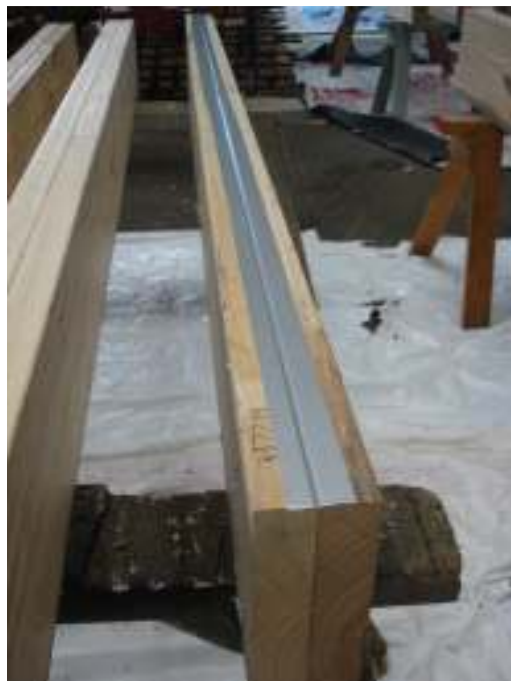
Figure 3: Cloth tape applied to under edge of lintel.
