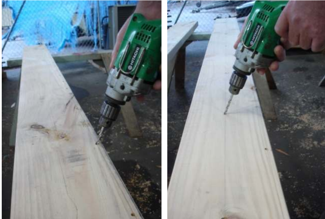
Figure 2: Drilling injection holes, single row of holes (photo on left) and double row of holes (photo on right shows hole at mid depth being drilled).
