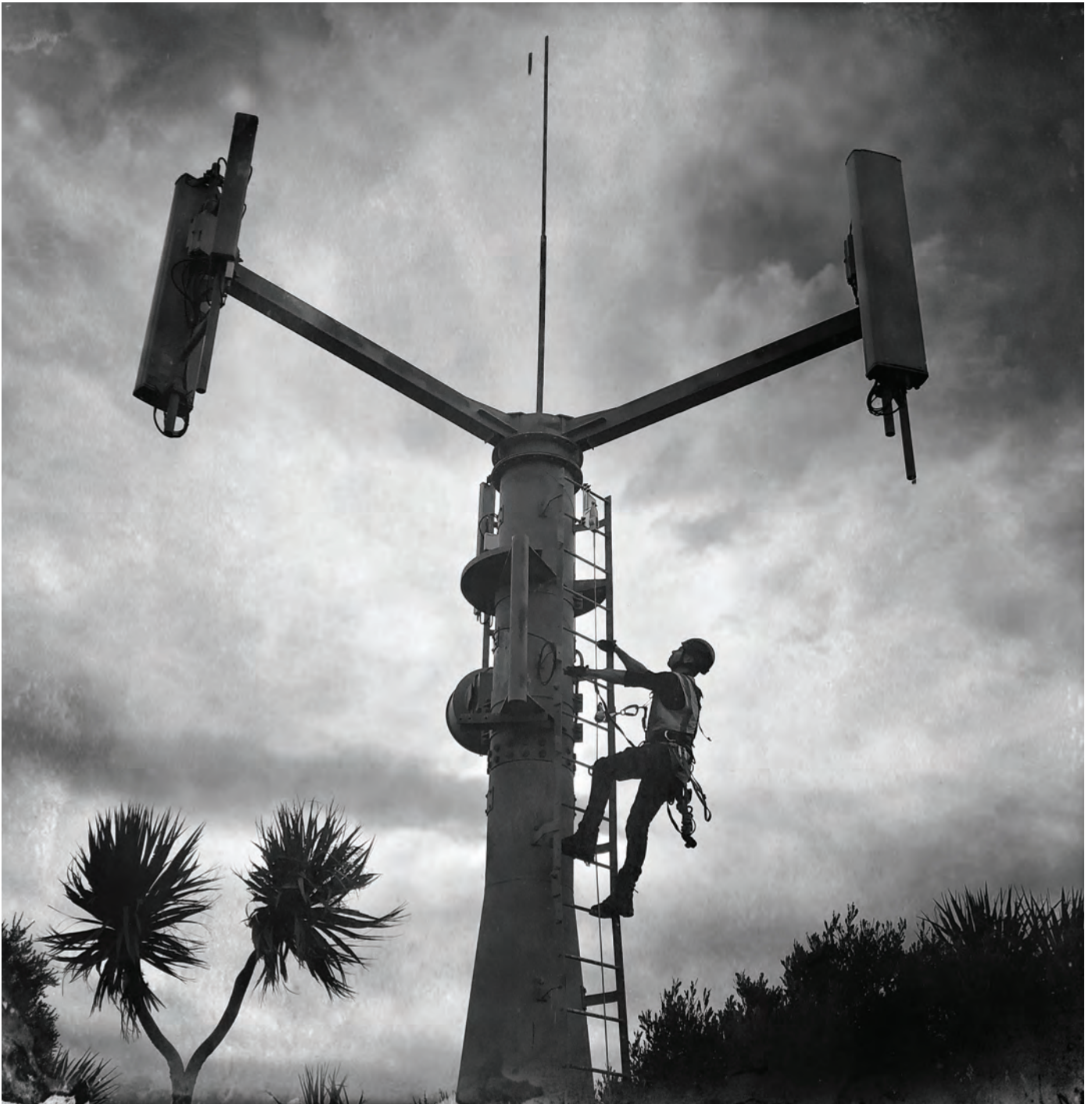
Cell tower. Haywards Hill, Upper Hutt
