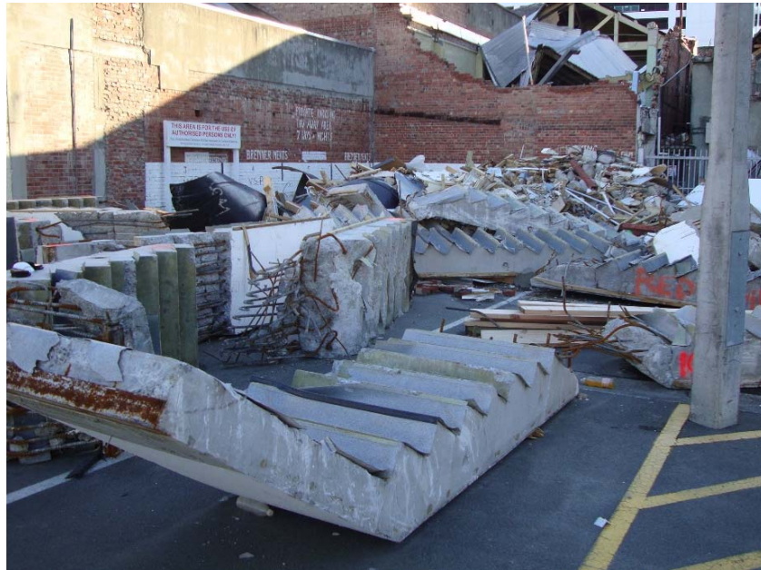
Figure 7.1 : Collapsed Stair Units Removed from Stairwell
