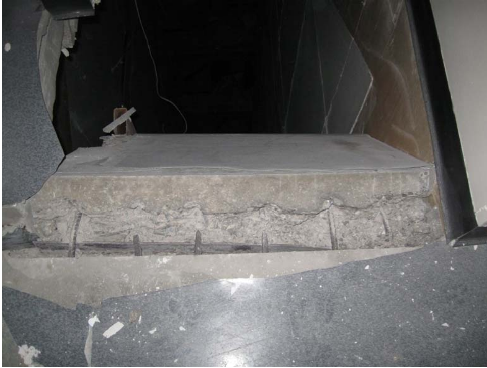
Figure 7.4 : Stair Flight Hanging from Top Starters (photograph taken from the top stair landing looking down the stair shaft).
