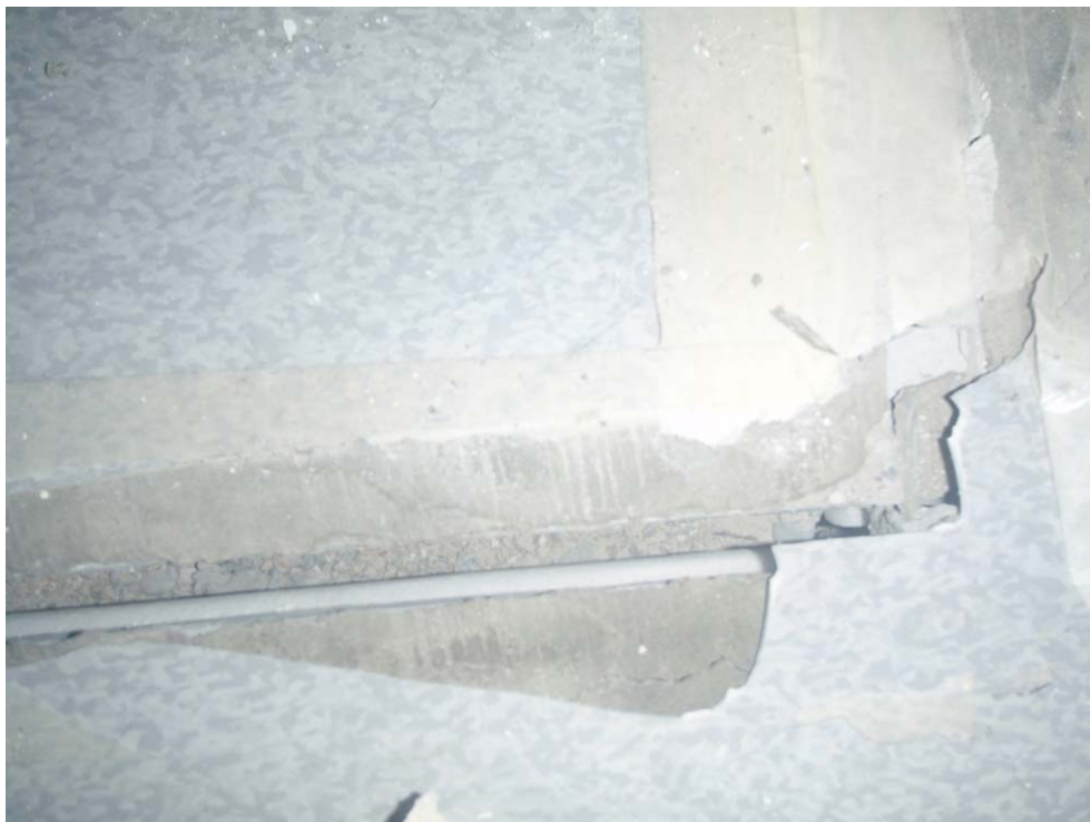
Figure 7.7 : Mortar-Filled Seismic Joint
