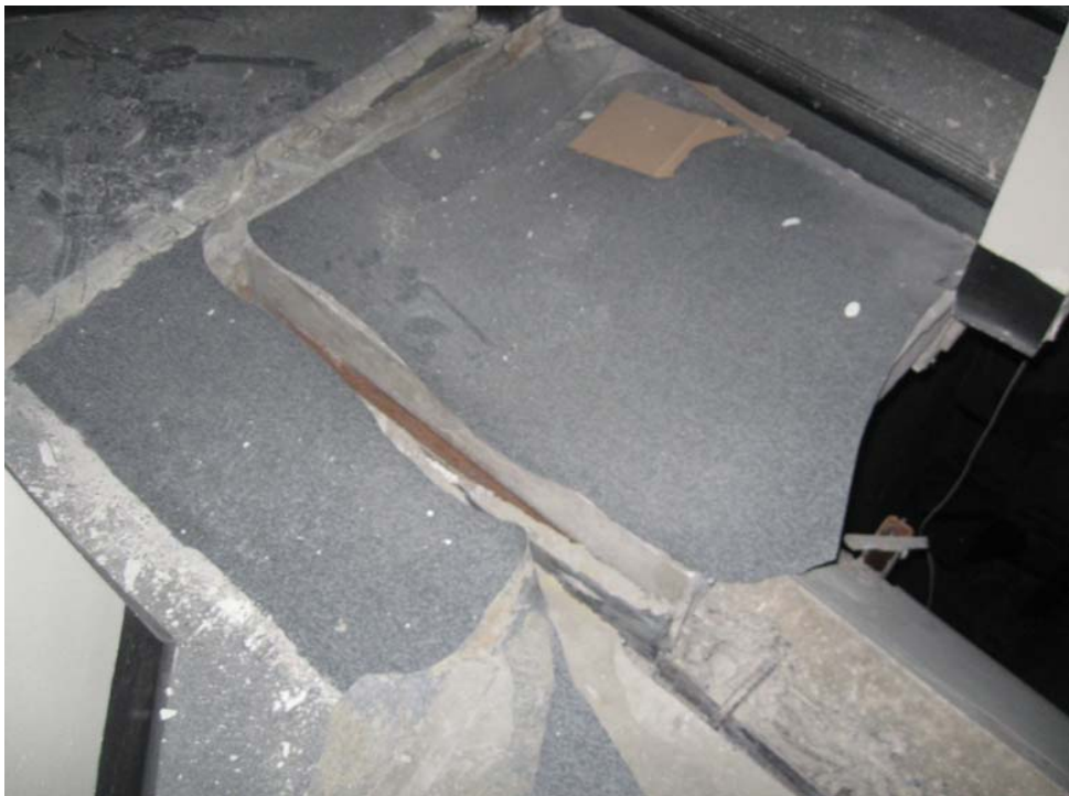
Figure 7.6 : Permanent Displacement at Bottom-Landing Seismic Joint
