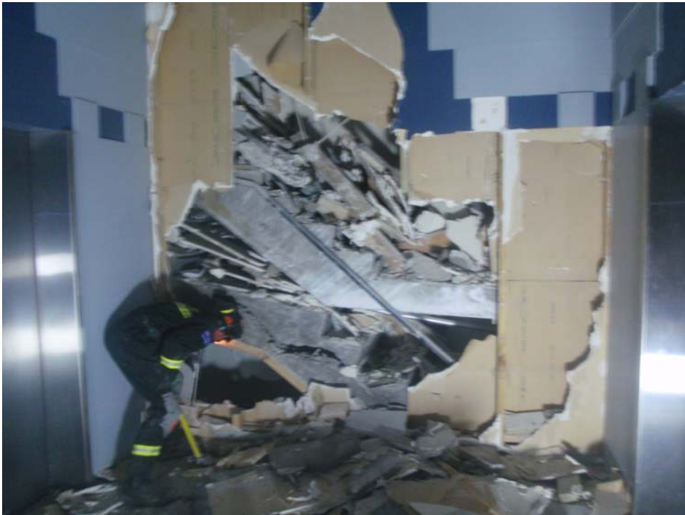
Figure 7.5 : Fallen Stair Flights at the Bottom of the Stairwell
