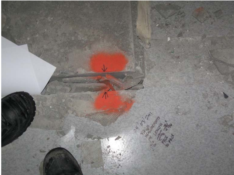
Figure 7.8 : Debris/Mortar in Displaced Seismic Joint
