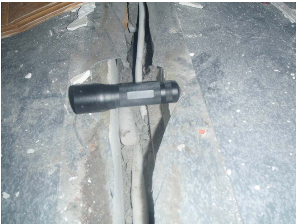
Figure 7.9 : Debris/Crushed Mortar below Sealant Backing-Rod
