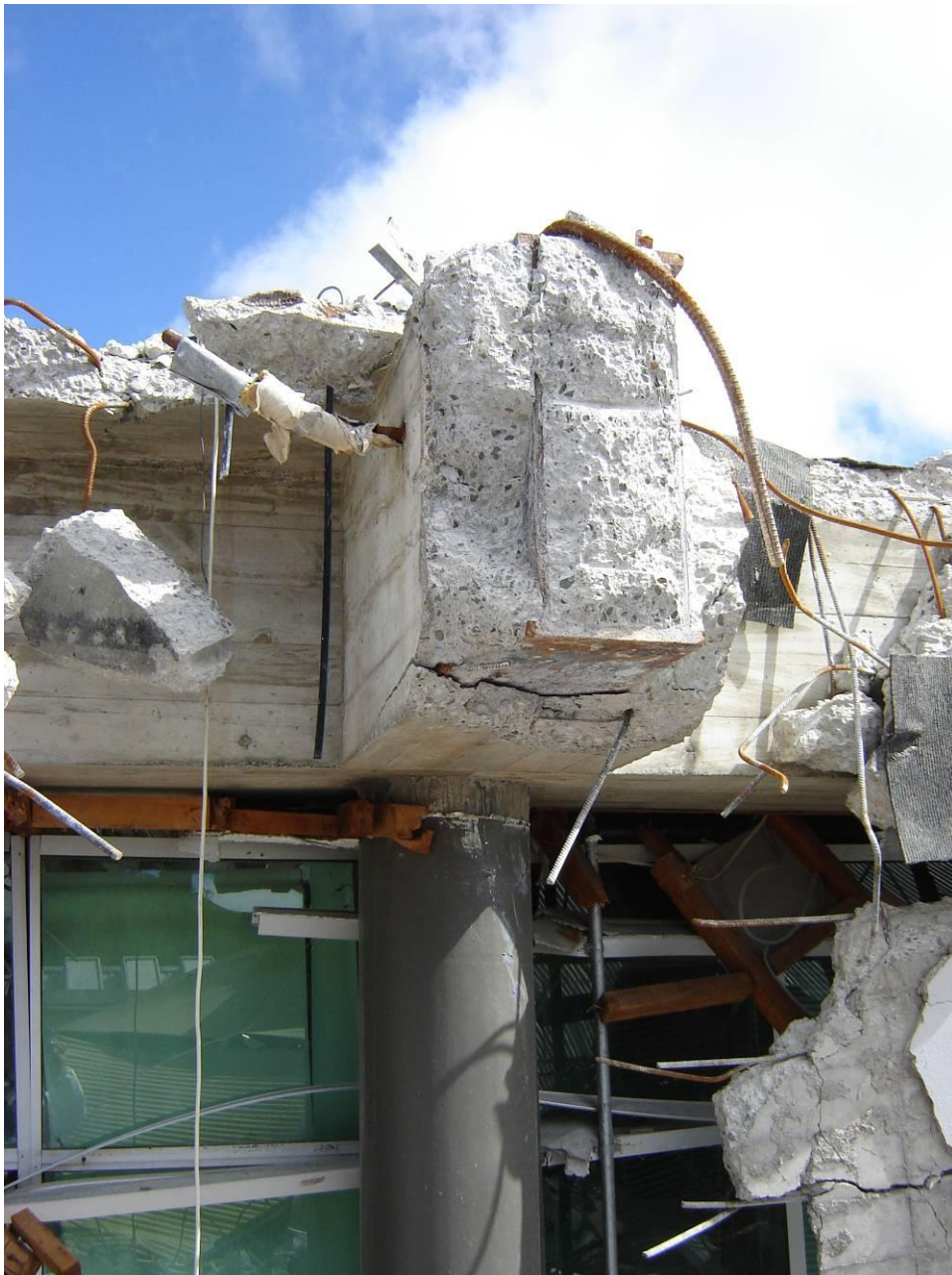
Figure 13 - Concrete Encased Steel Girder on Steel Jacketed Concrete Column
