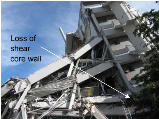
ex USAR engineers
