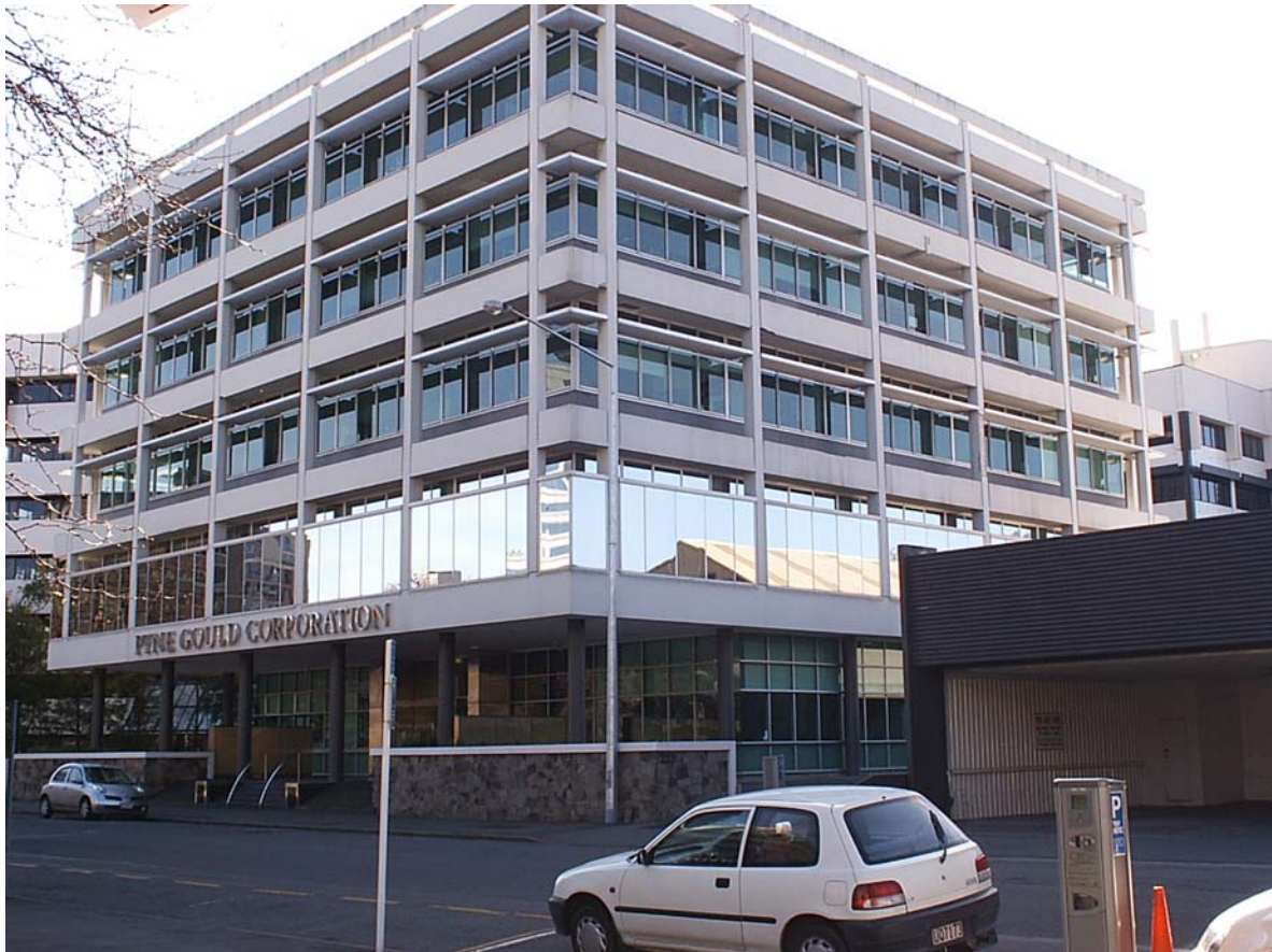
Figure 4.1 : 2010 Photo of Building taken from South-East
