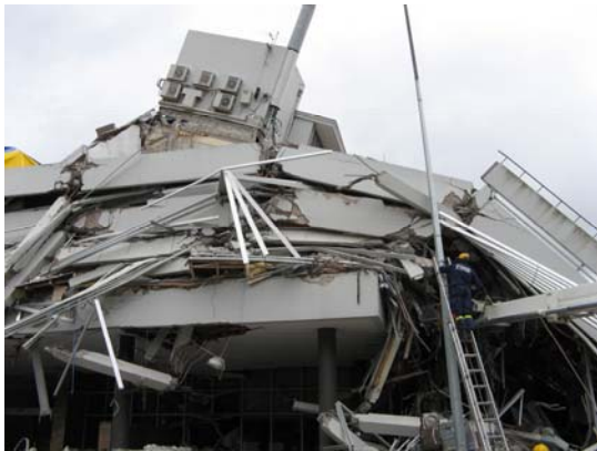
ex USAR engineers
