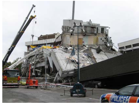
ex USAR engineers
