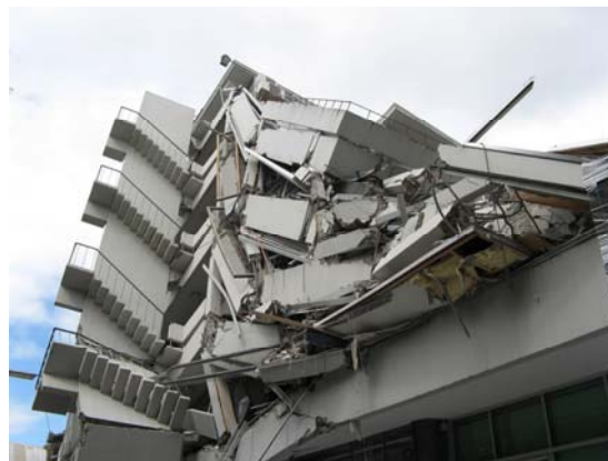
ex USAR engineers
