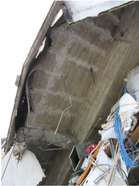
ex USAR engineers
