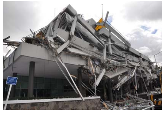
ex USAR engineers
