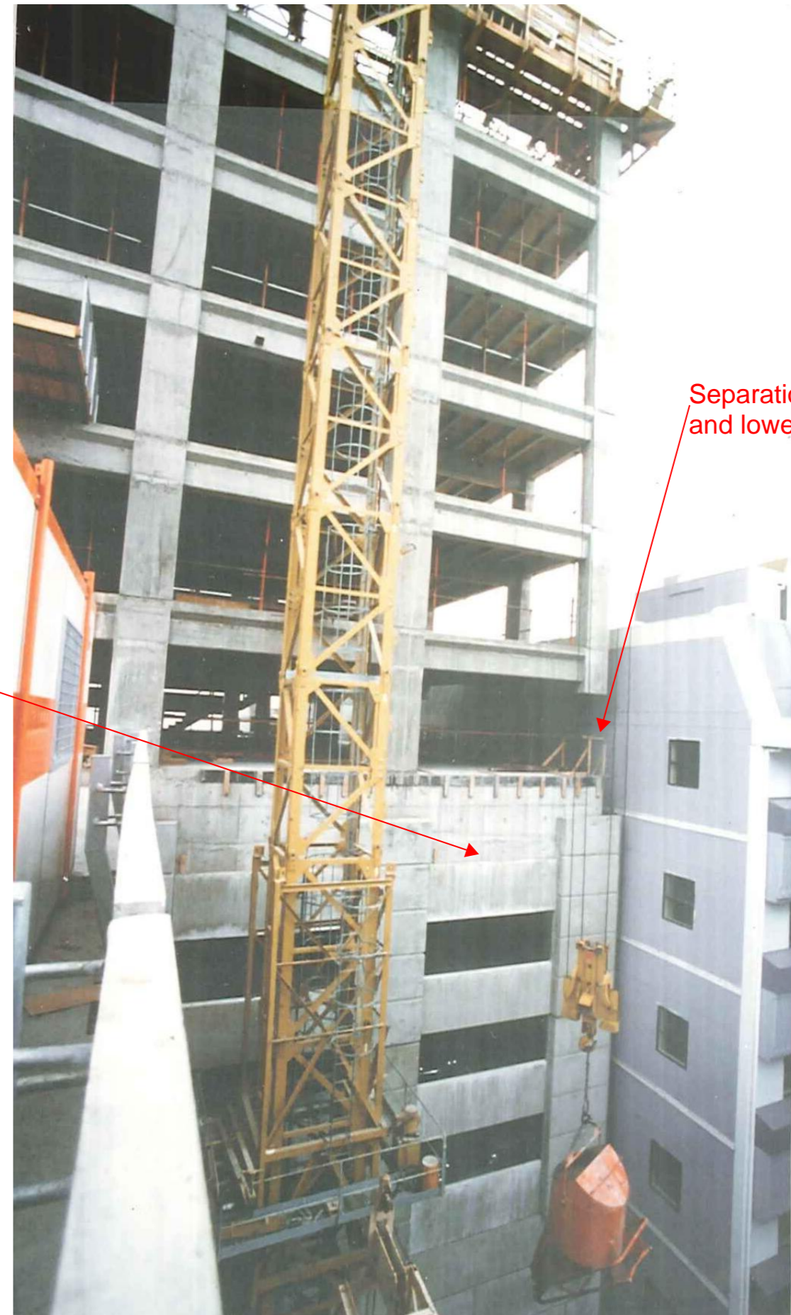
Photo 2 - Southern Elevation - During Construction
