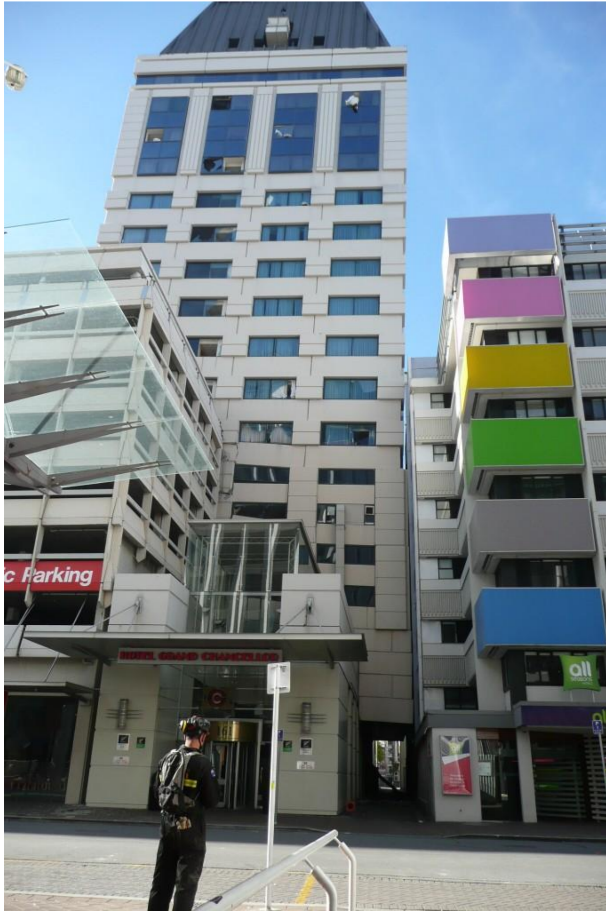
Photo 3 - Southern Elevation - Post February
