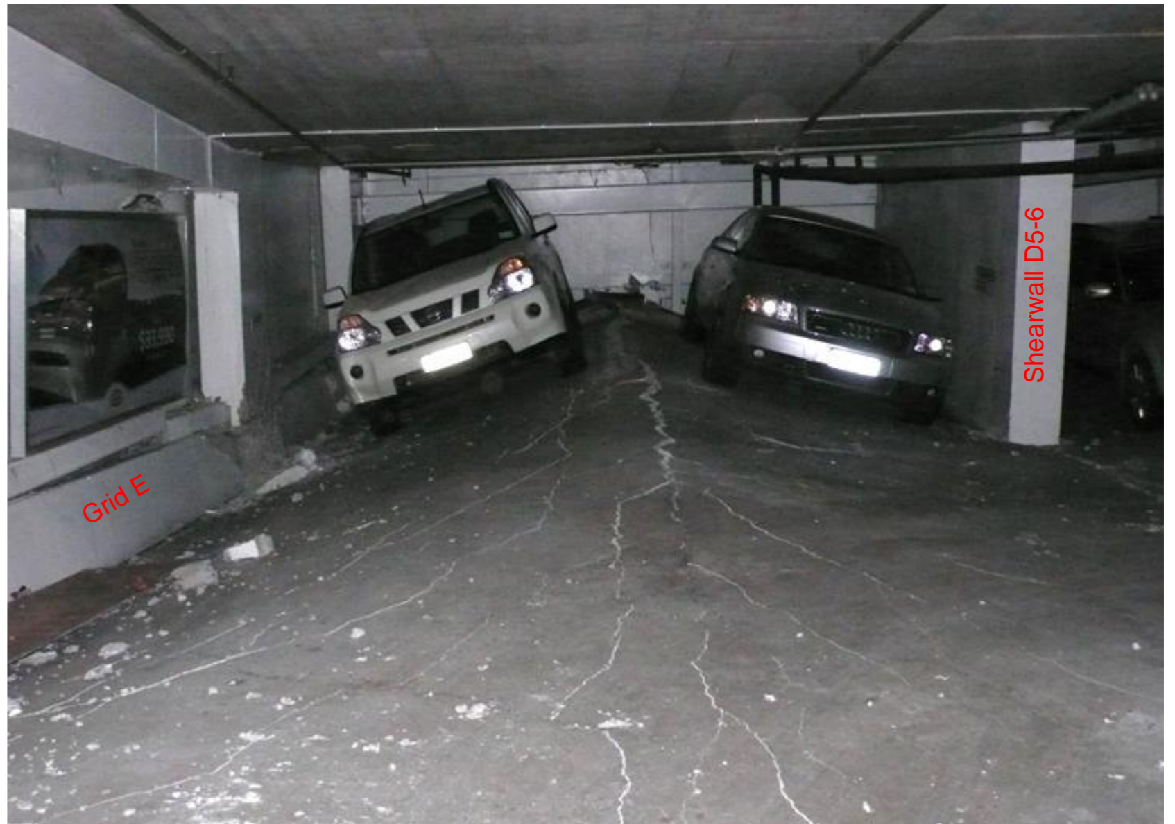
Photo 13 - Folded slab at level 2
