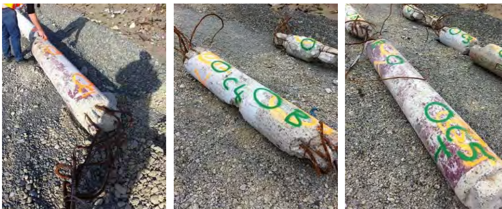
Figure 49 -400 mm diameter columns full height (left to right) (a) Test Item tC1 Level 6 to roof column with base hinging failure, still connected by reinforcing to tC8 below; (b) tC4 hinging top and bottom; (c) tC5 Level 6 to roof column with hinging at base.
