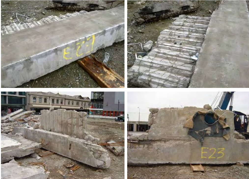
Figure 8 - Edge Shell Beam (Item E23) from Line 1 or 5. (Clockwise from top left) (a) Underside and outer face; (b) Underside showing 1200 mm slab outstand with metal decking pulled away and diagonal cracking indicating shear in diaphragm; Holes are where concrete cores were taken for testing; (c) Carpet remnant on top of slab; (d) Damaged shell beam.
