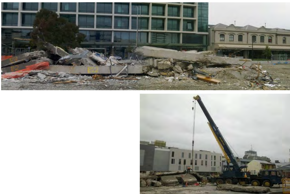
Figure 3 – Structural debris pile on CTV site (top to bottom) (a) At start of Site Examination; (b) Crane used to move debris remnants for examination
