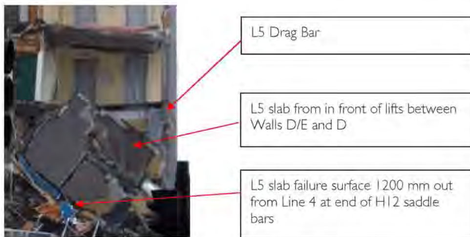
Figure I 64 - Level 5 slab from in front of lifts shortly after the collapse.
