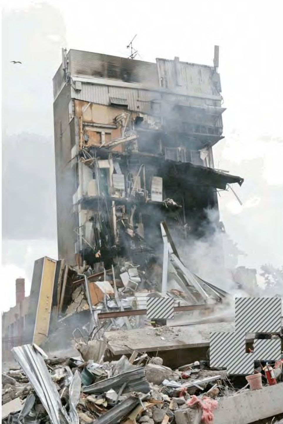
Figure 82 - Spandrel Panels and beams at Cashel Street Line 1 and on Line 4 in background standing vertical. Roof steelwork debris is visible.
