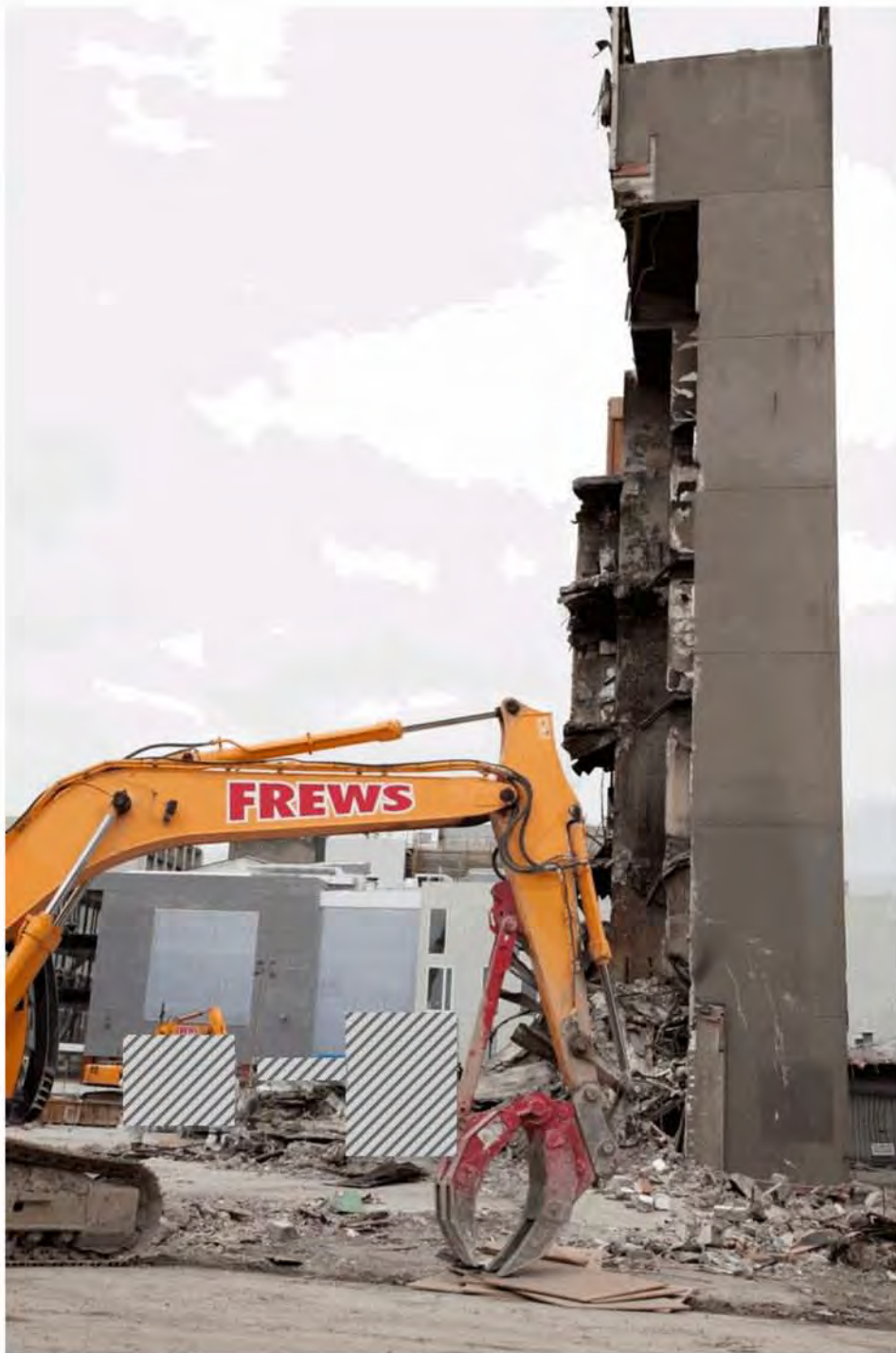
Figure 103 - North Core slabs removed.
