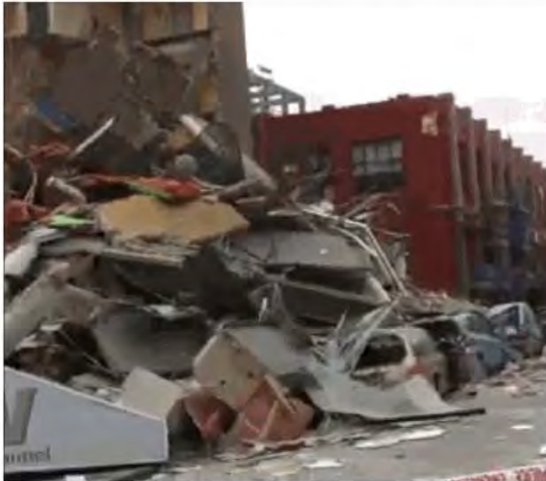
Figure 78 – View from southeast corner of CTV Building along Madras Street. This shows Line F Spandrel Panels fallen onto cars parked in the street indicating a tilt to the east during collapse.
