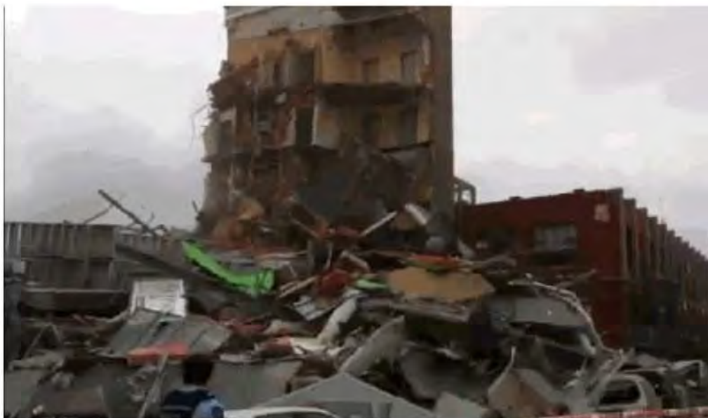
Figure 76 Madras St with precast Spandrel Panels fallen onto cars.
