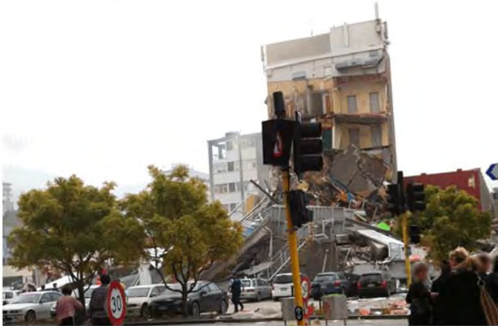
Figure 73 - Cashel St. face with North Core tower in background prior to fire starting.
