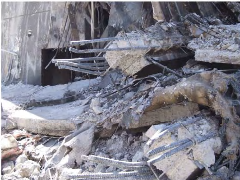
Figure 99 - Line 3 beams lying rotated southwards
