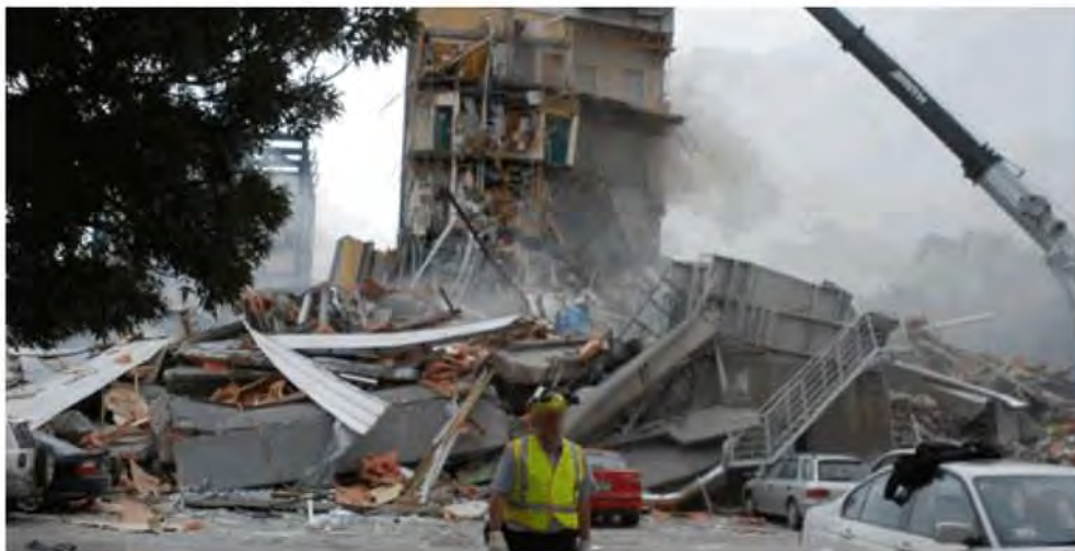
Figure 74 - Western end of south face (Line 1). Collapsed Line shear wall with escape stair to the right.
