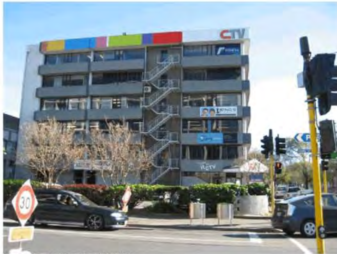
Photo 1 South Elevation of Building
