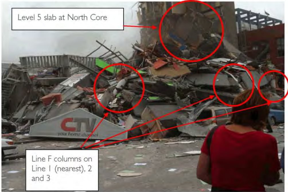
Figure 77 - Corner of Cashel and Madras Streets looking towards North Core. Fractured columns and fallen Spandrel Panels are visible (MSN photo).
