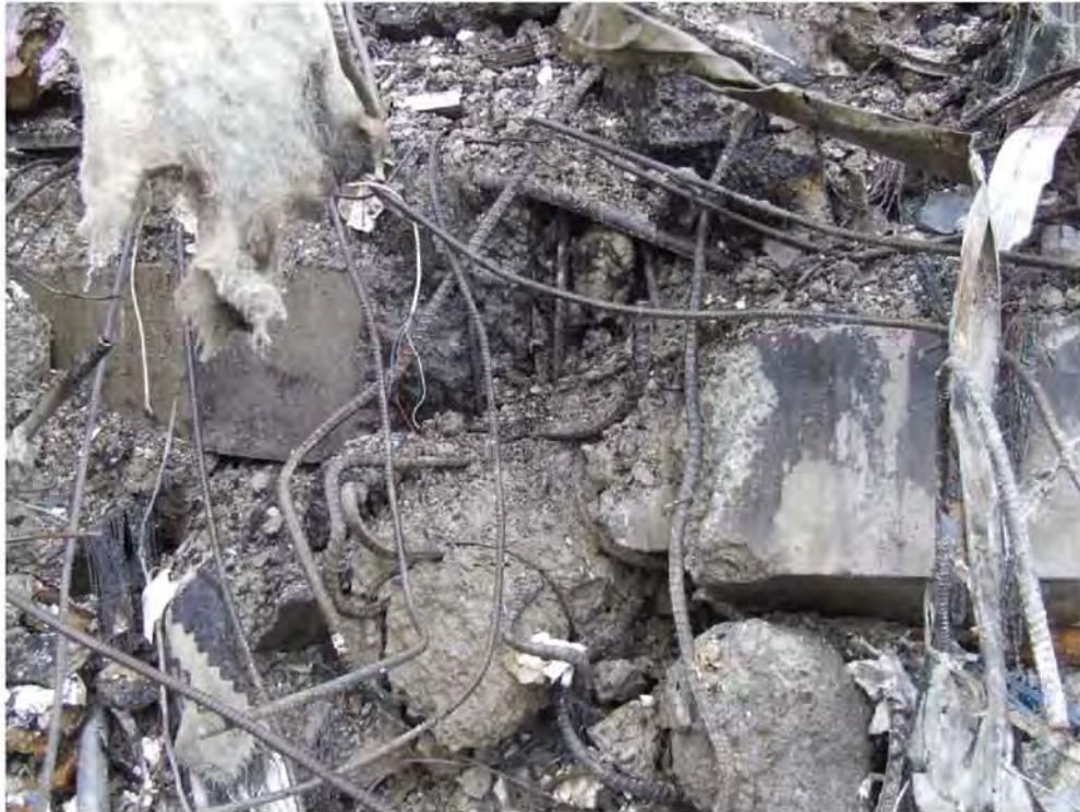
Figure 100 - Perimeter columns at beam-column joint with shell beam on right side.
