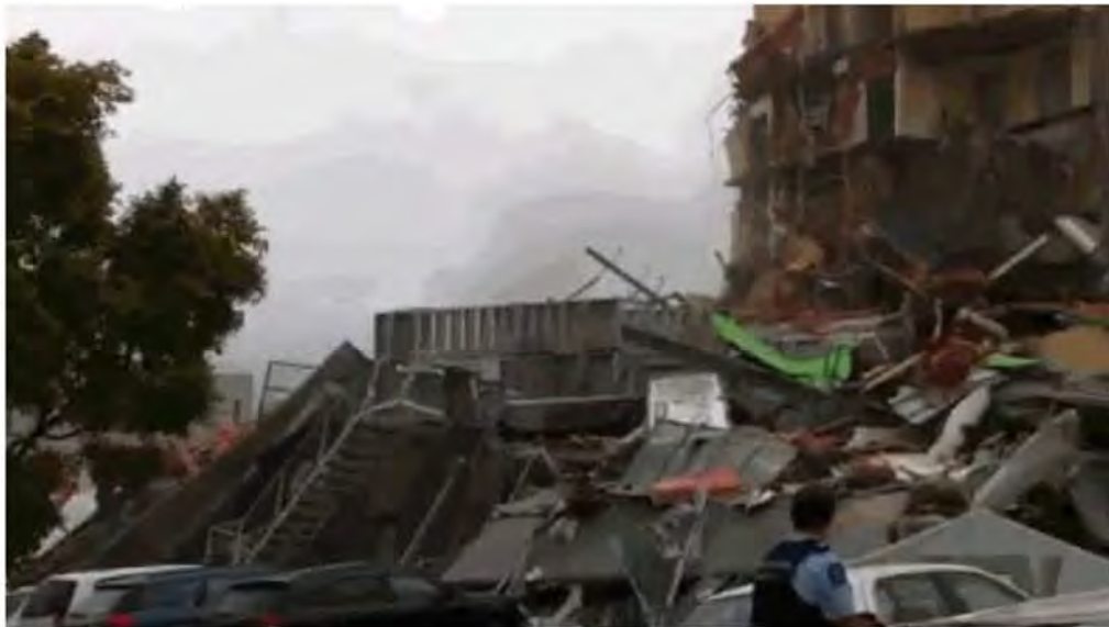
Figure 75 – View southeast corner of the CTV Building looking northwest. The South Wall collapsed onto the top of the debris from Level 2 can be seen, identifiable by the white fire escape stair still attached to it.
