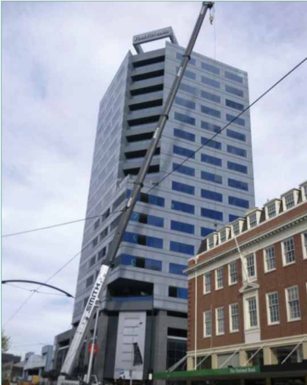
Figure 8.1: The Forsyth Barr Building from Armagh Street (looking south-east)
