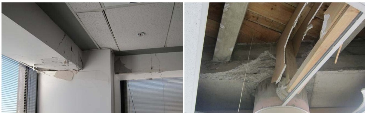
Figure 36: Post-1970s reinforced concrete moment-resisting frame buildings collapse/damage patterns: a) Two-way plastic hinging on 5 th floor of a 22-storey office tower; b) 2 nd floor beam-column connection in a five-storey office building
