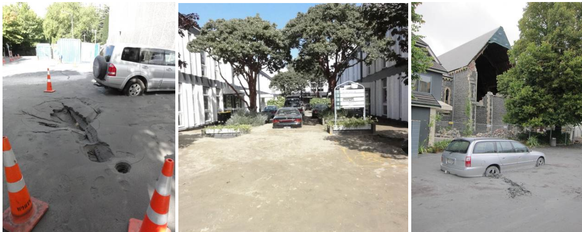
Figure 19: Liquefaction damage within the Christchurch CBD: a) Kilmore Street ; b) Armagh Street ; c) Manchester Street
