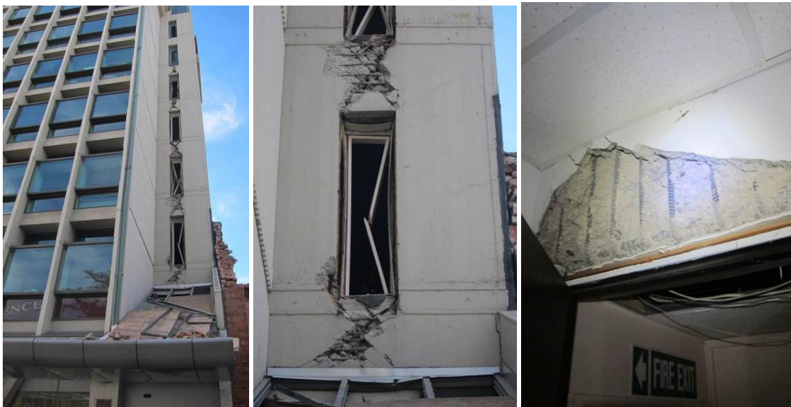
Figure 40: Pre-1970s reinforced concrete structural wall buildings collapse/damage patterns: a-b) Seven-storey 1960s coupled-RC walls building with significant damage on the coupling beams. Plain bars and diagonal reinforcements were used on the coupling beams; c) Six-storey 1950s RC walls building with moderate damage to the coupling beams
