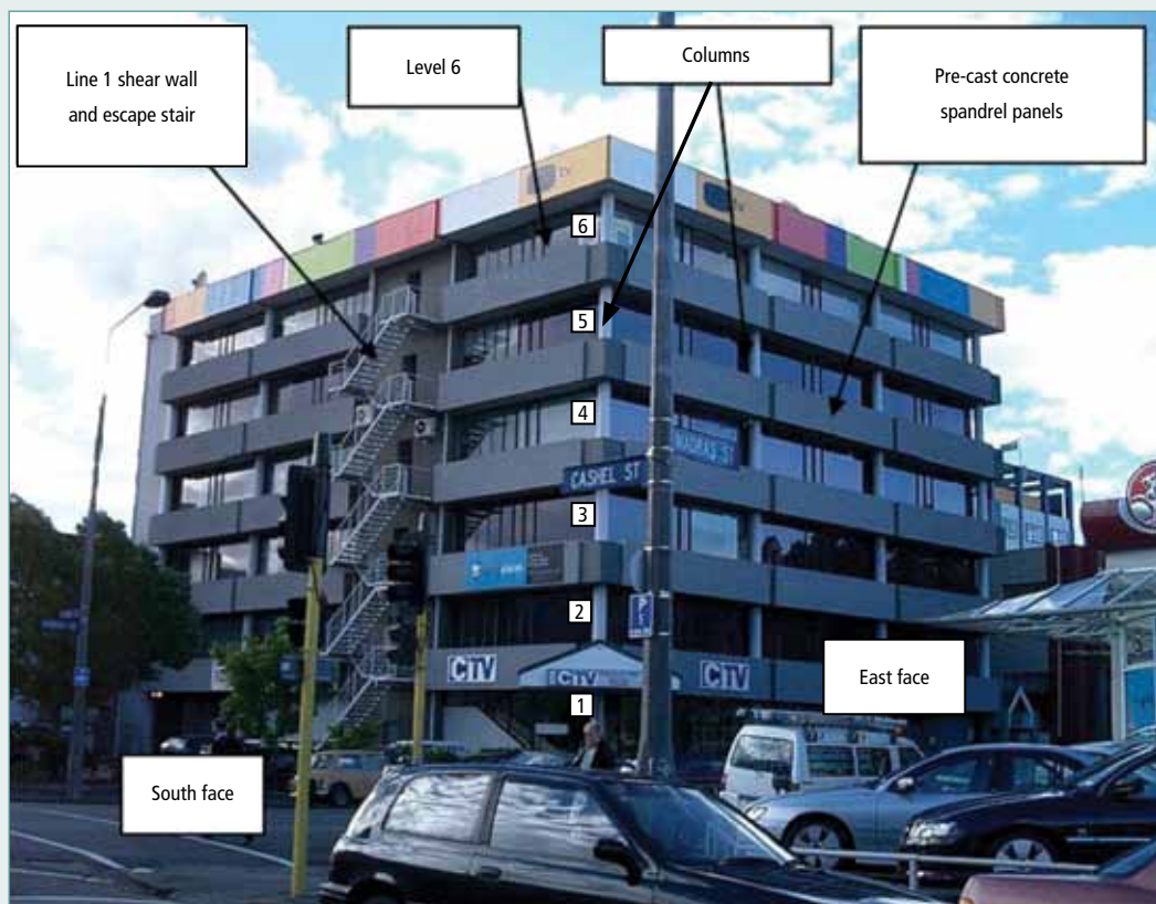
Figure 5.1: Canterbury Television Building in 2004 (Photo credits: Phillip Pearson, derivative work: Schewede66)
