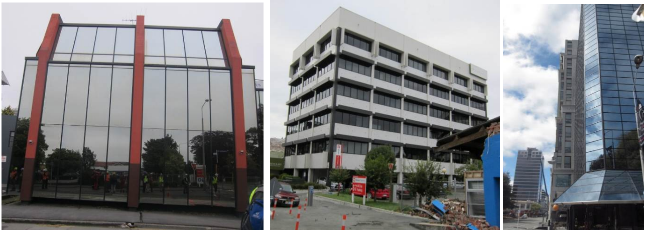
Figure 20: Liquefaction induced differential settlement resulting in significant tilting of mid- to high-rise buildings of various foundation and soil details: a) Four-storey with shallow foundation; b) Six-storey with piled foundation; c) Three high-rise buildings with substantial differential settlement and tilting.
