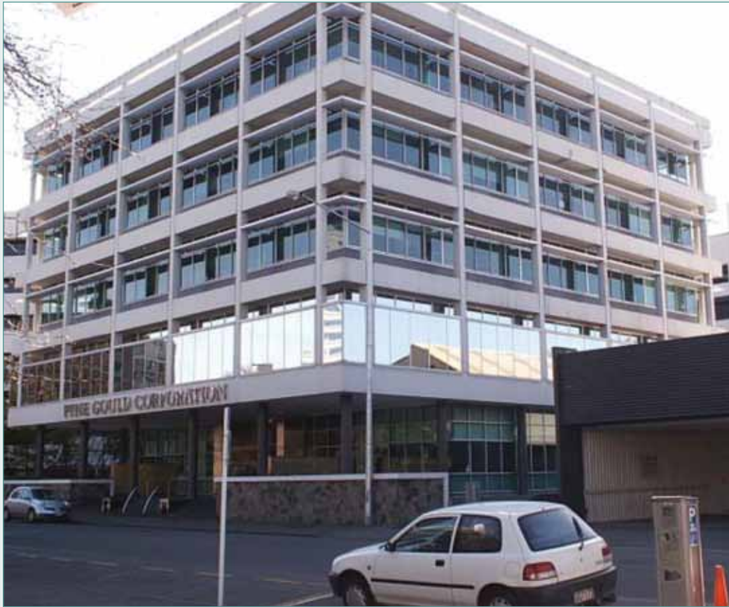
Figure 6.1: PGC Building prior to collapse (source: S. Tasligedik)
